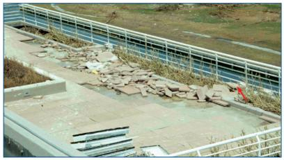
Figure 1 – View of lifted pavers on the fifth floor roof. The red arrow indicates a paver resting on the top of the parapet.
